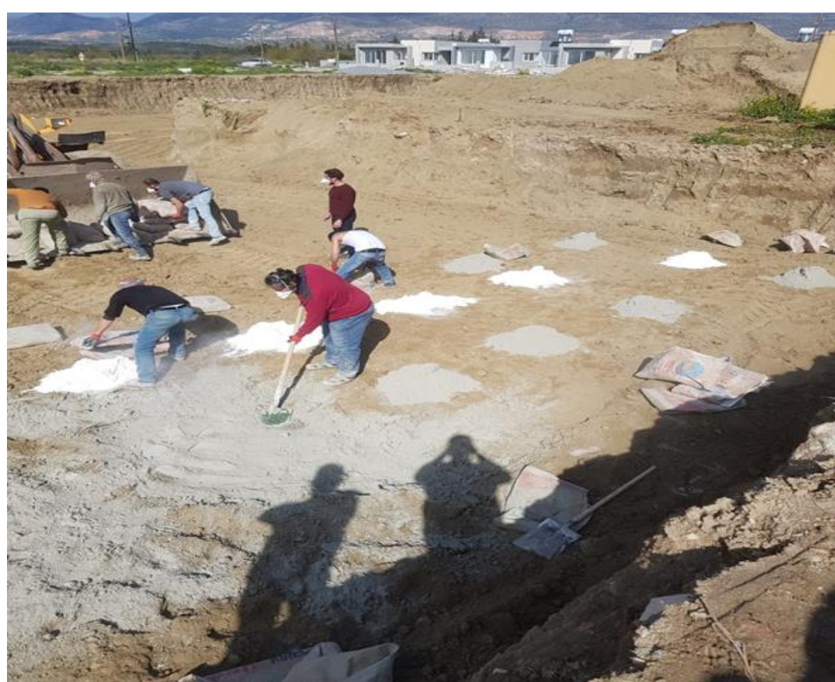
Demonstrates Spreading of Cement by Workers
